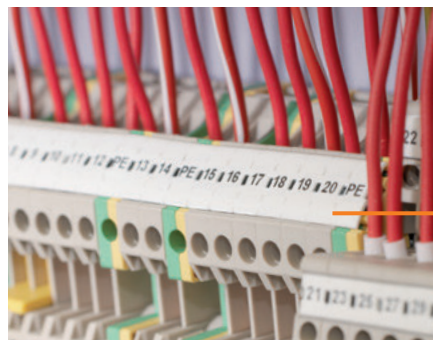
DEK/WS: Flexible connector markers - print, clip, finished
